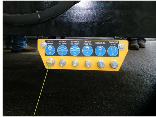
4-WAY VALVE GREASE POINT
