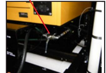
Tank Cleanout Valve
