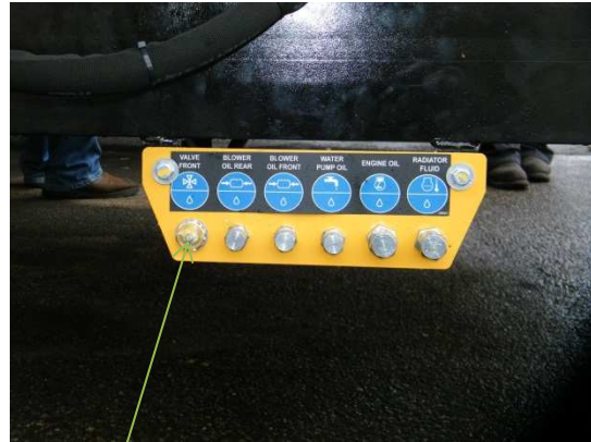
4-WAY VALVE GREASE POINT
