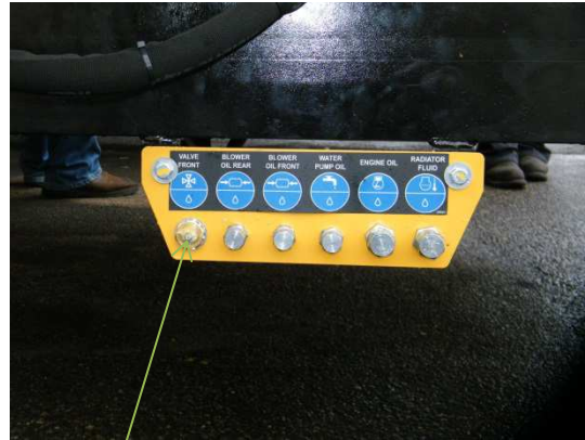
4-WAY VALVE GREASE POINT
