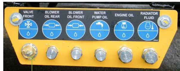
4-WAY VALVE GREASE POINT
